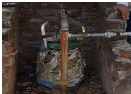
Bore well at Chanch Village
